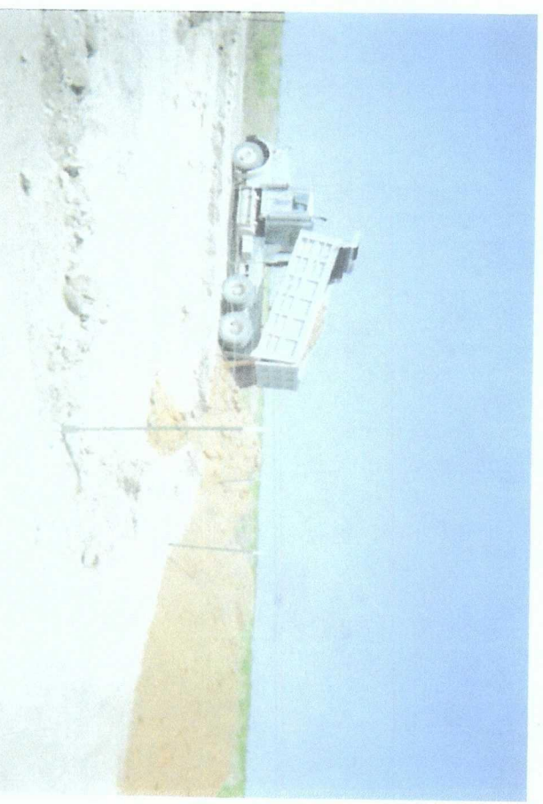
clean, imported dirt being unloaded; facing west
