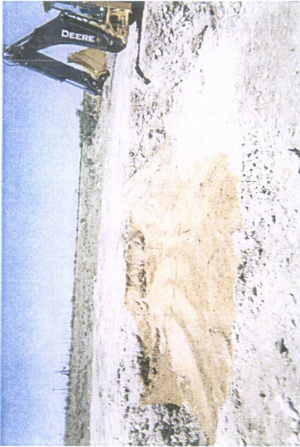
clean, imported blow sand used as padding below the liner, facing north
