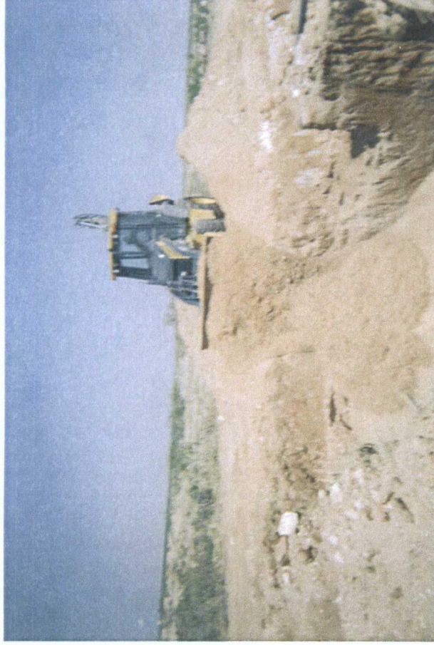
backfilling excavation
