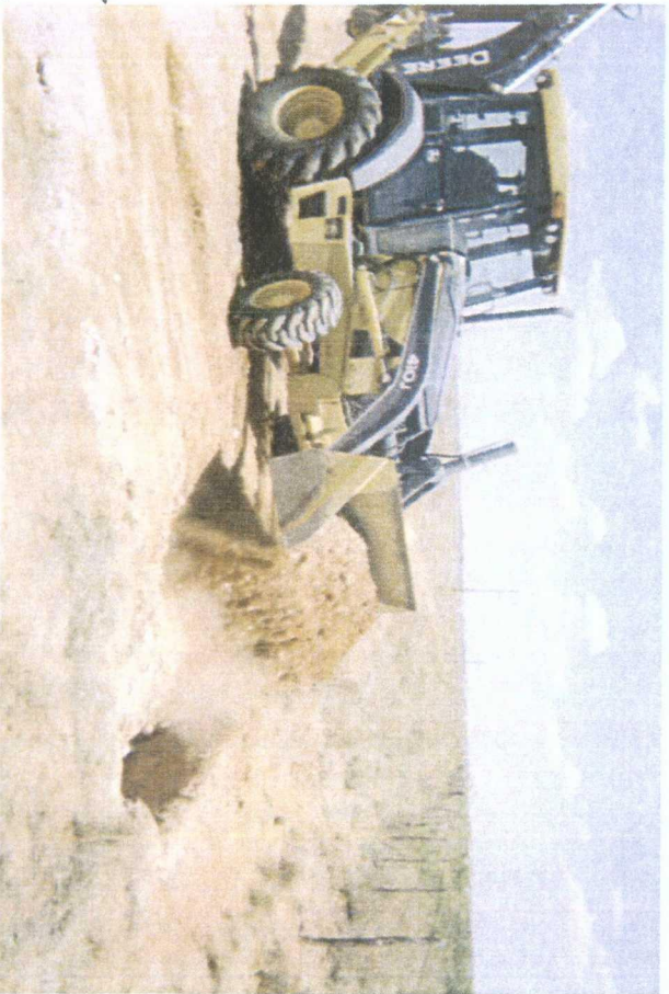
backfilling excavation
