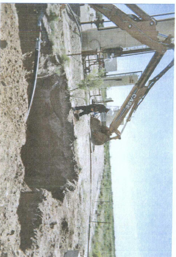
collecting soil samples from the trench
