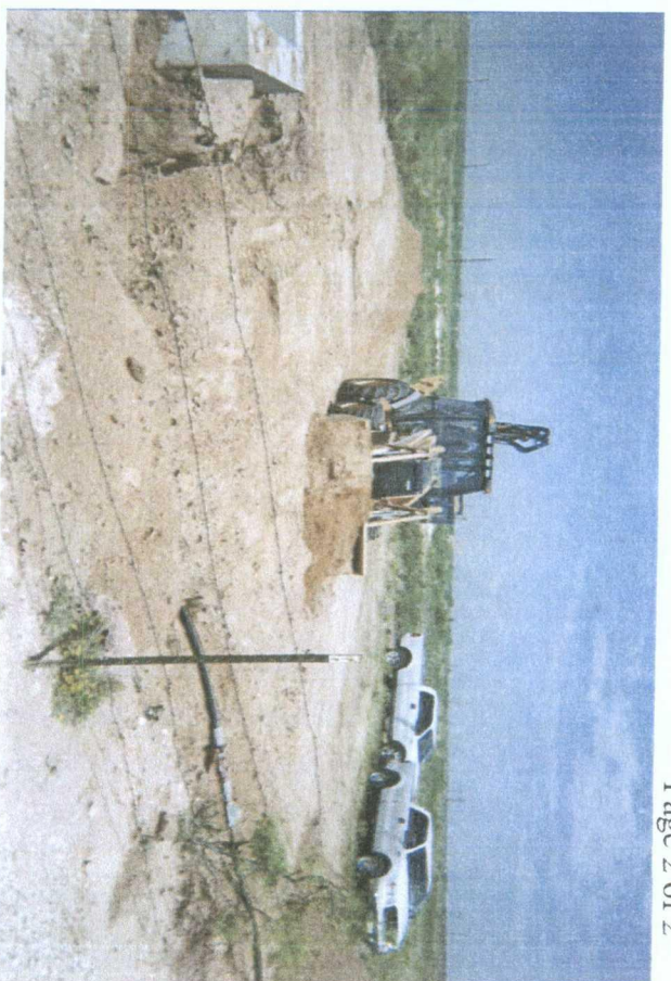
spreading clean, imported soil
