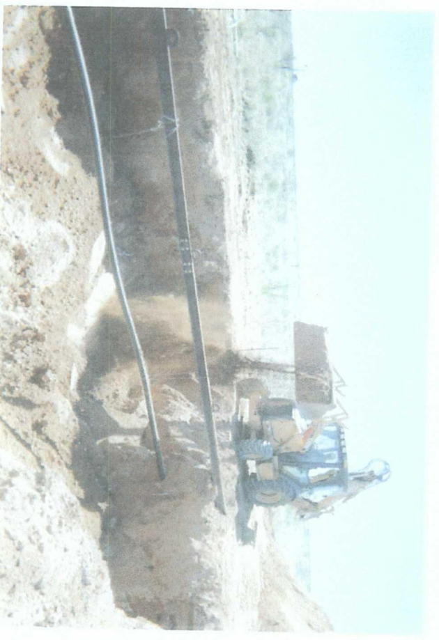
backfilling excavation up to 6 ft BGS
