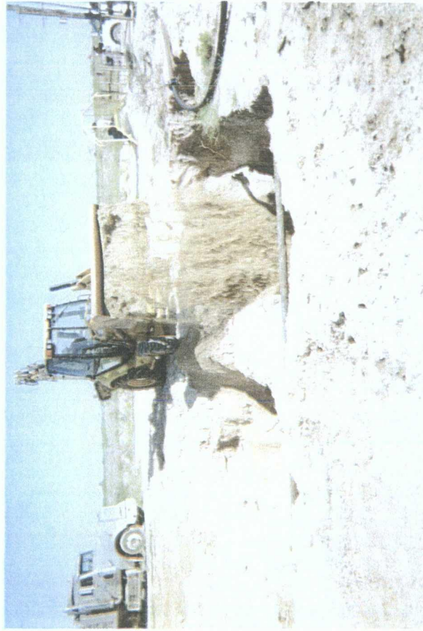
backfilling the 20x20x12-ft excavation
