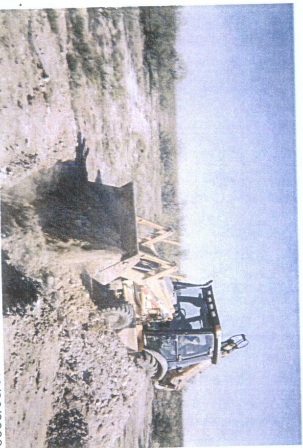
backfilling excavation
