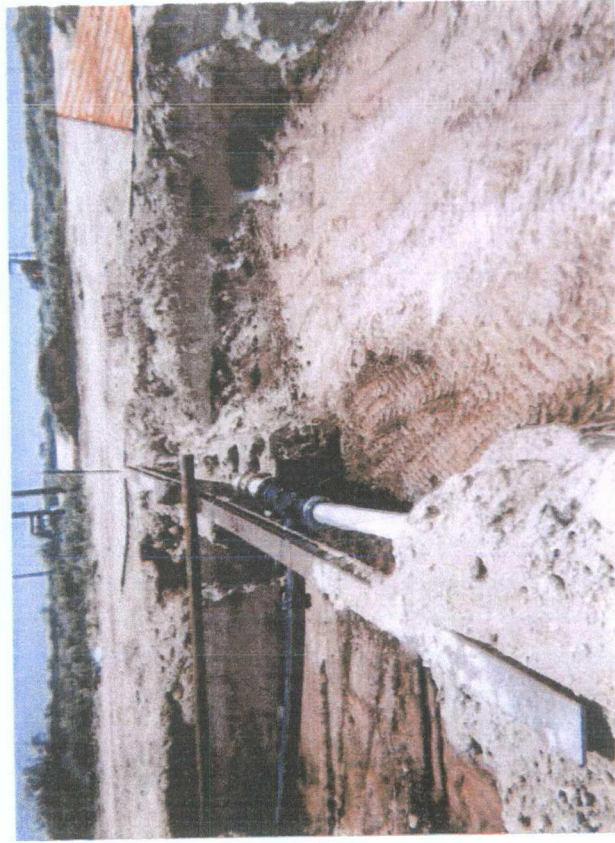
clay barrier installed
