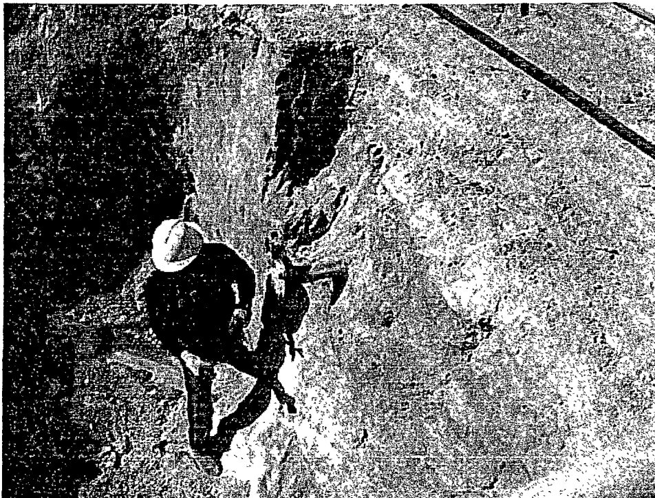
Capping the former pipe connection.
