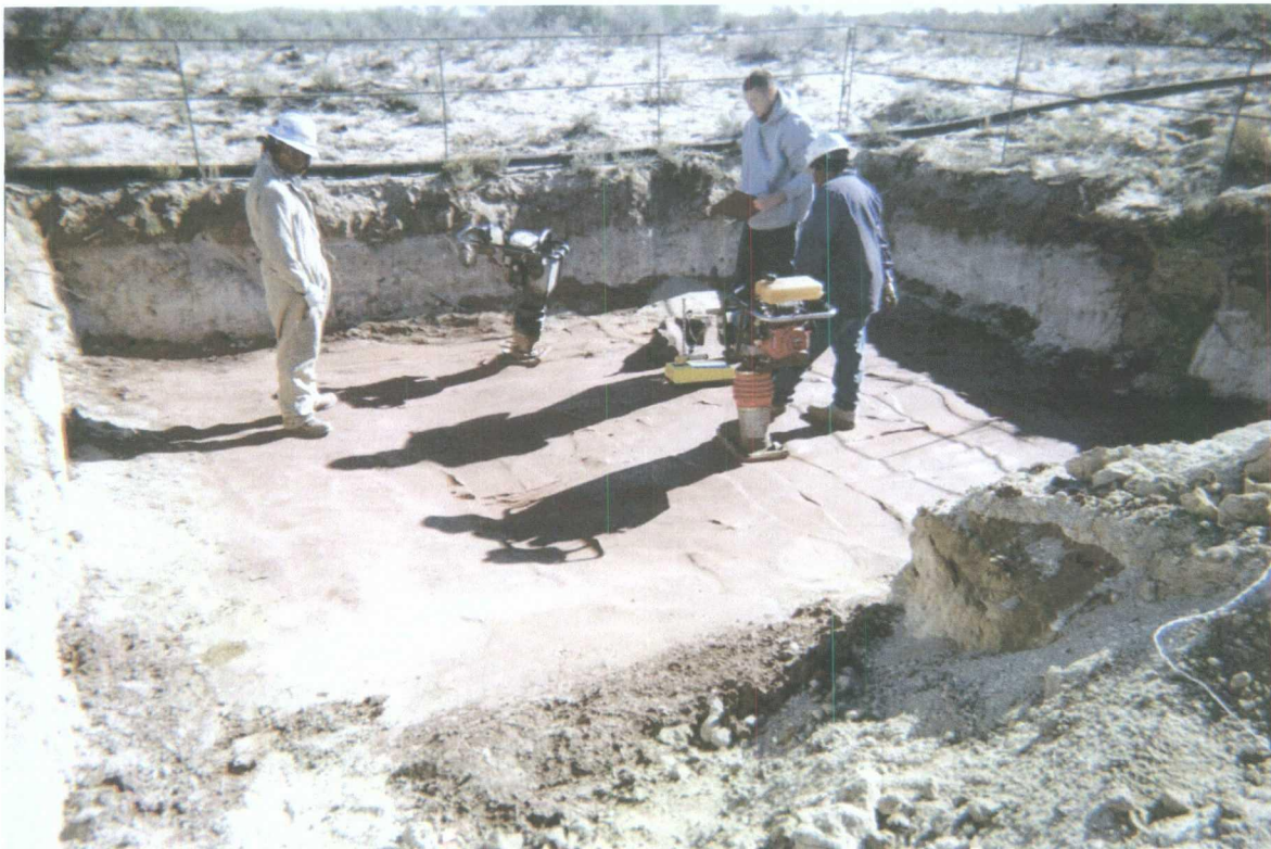
Figure 4 – Installation and compaction of subsurface clay barrier at EME State H EOL.
