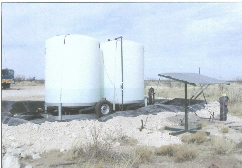
Figure 3 – Vac N-6-1 solar-powered groundwater recovery system.
