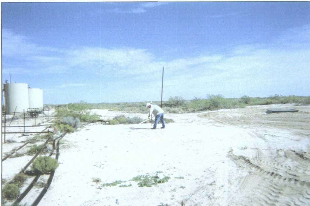
Figure 10 – Raking and seeding of reclaimed site.
