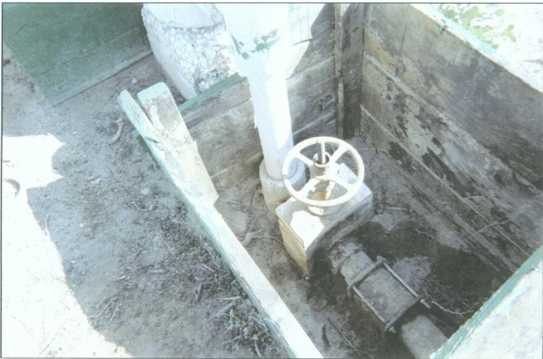
Figure 7 – Former junction box before removal, close-up view.
