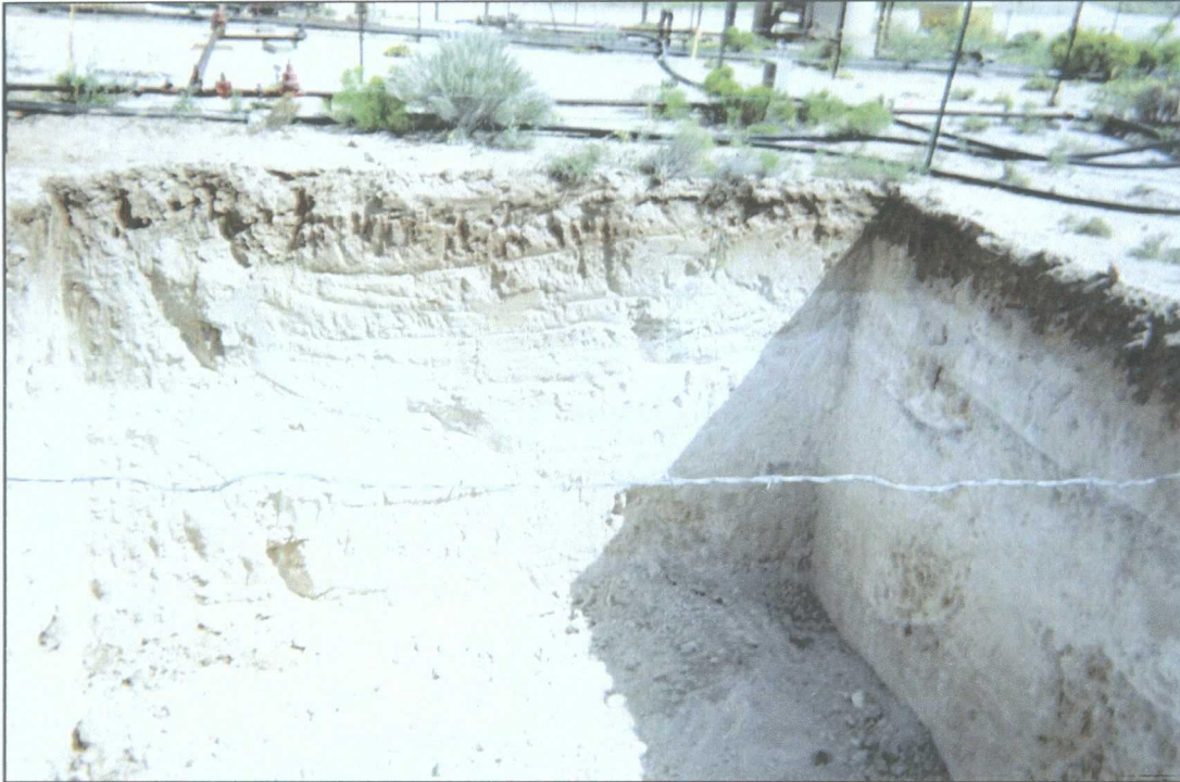
Figure 8 – Excavation following removal of former junction box.
