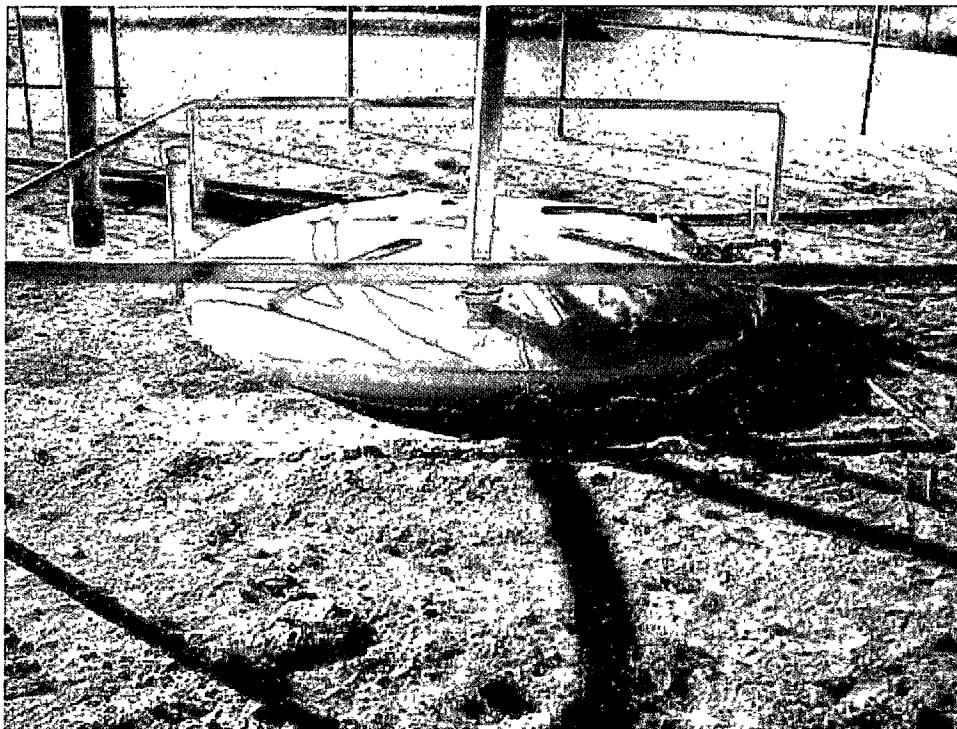
Below-grade tank prior to closure.
