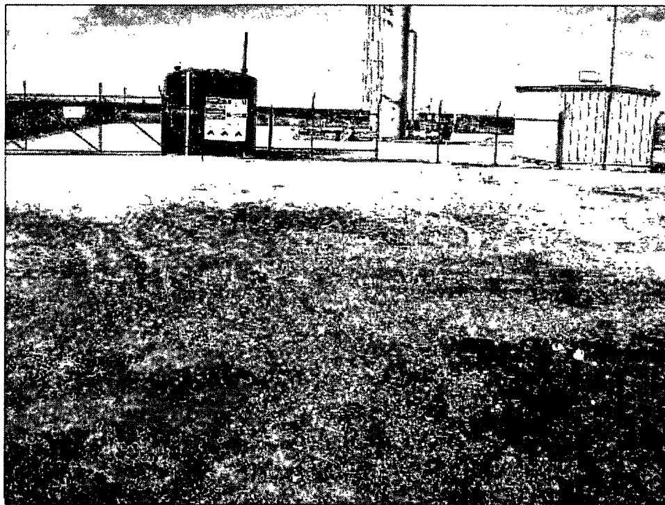
Top soil placed as final fill lift. Tank closure is considered complete.
