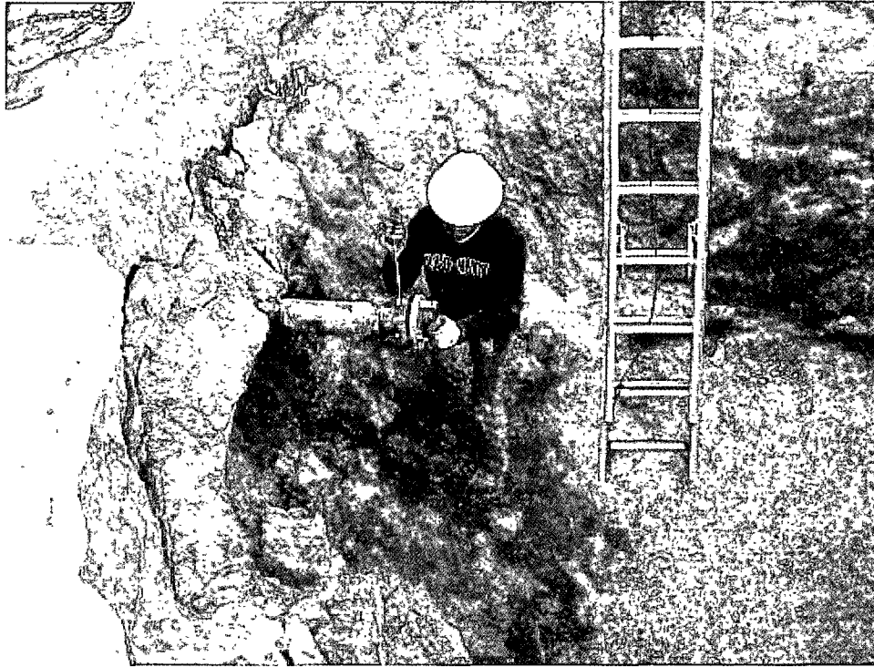
Installing a Slip Plate Cover over discharge line
