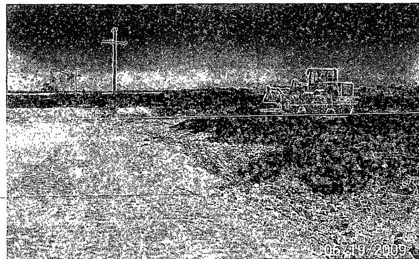
Photo #34 Backfilling of Excavated Area
