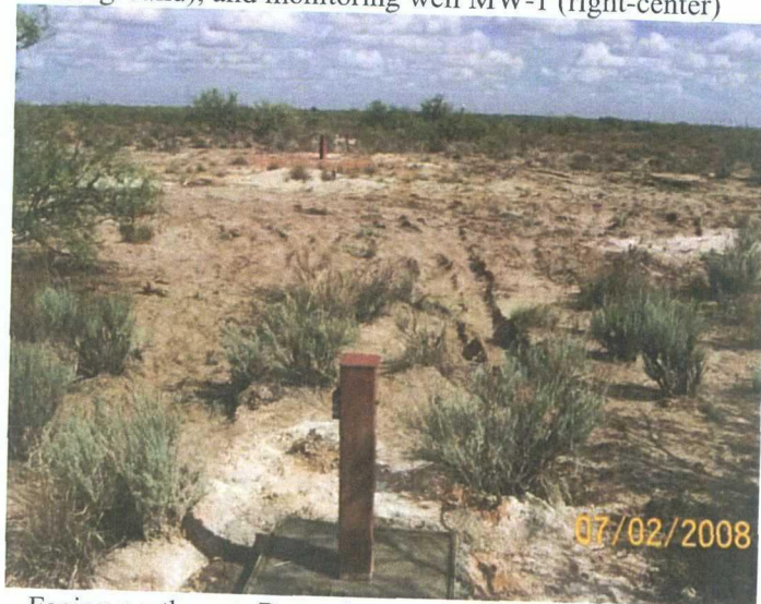
Facing northwest: Recently completed monitoring wells MW-3 (foreground) and MW-1 (background)
