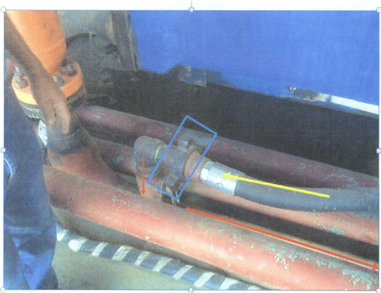
The picture below shows the inlet to the wellhead. The red line is the line coming from the pumps and is the line that will be pressure tested. The valve designated with the yellow line will be closed to maintain the pressure in the discharge line.
