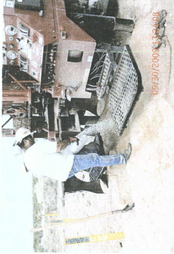
plugging SB #1 with bentonite
