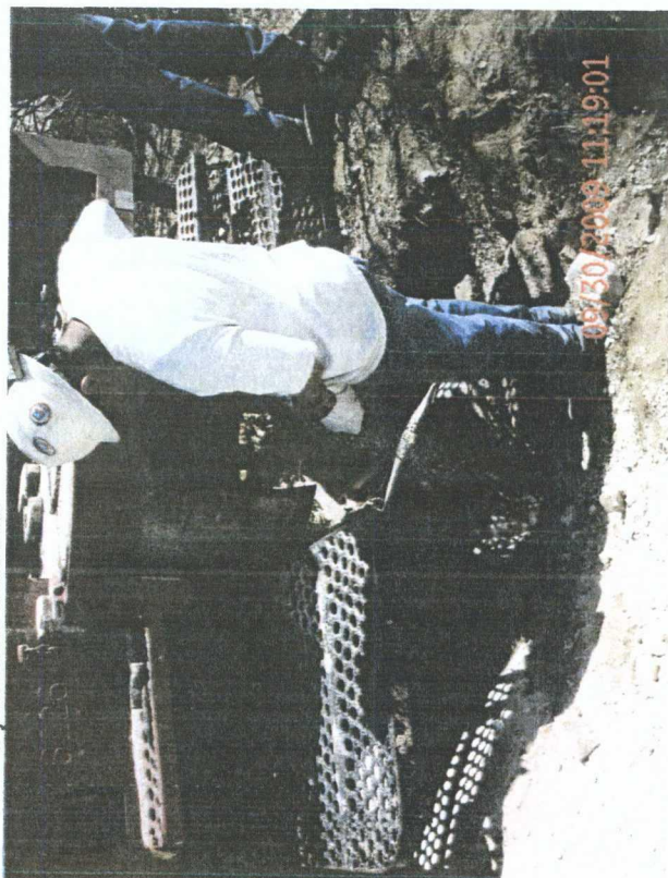
drilling the soil bore at the former junction box site 9/30/2009
