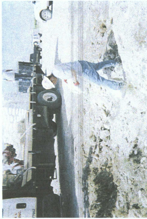
plugging SB #1 with bentonite
