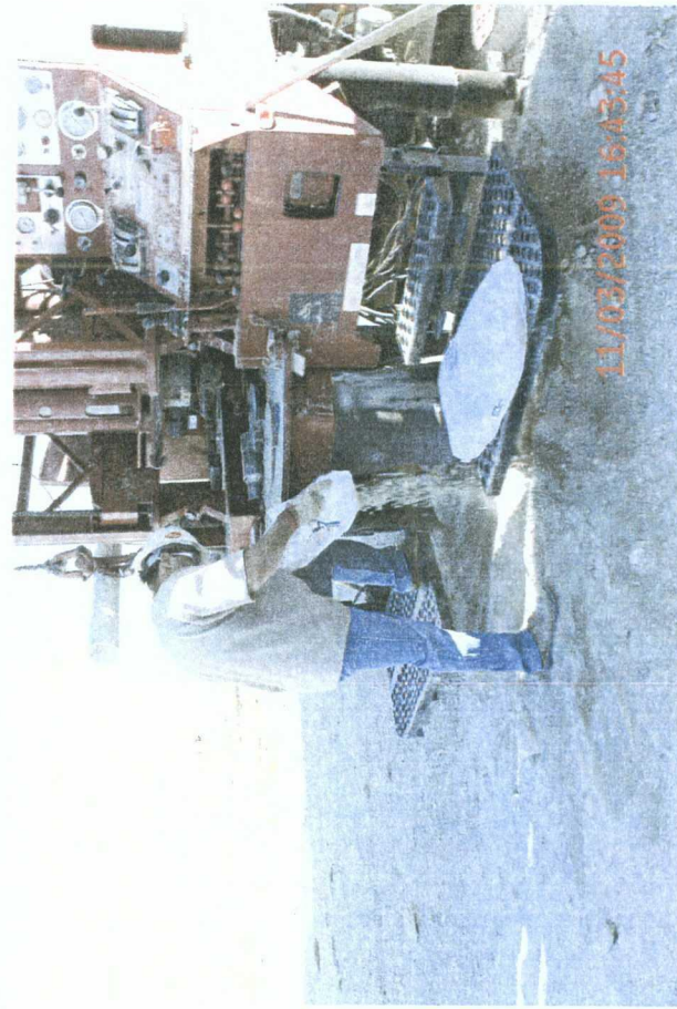
plugging SB #1 with bentonite
