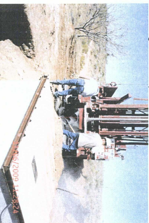
drilling SB #1 and the new, watertight junction box
