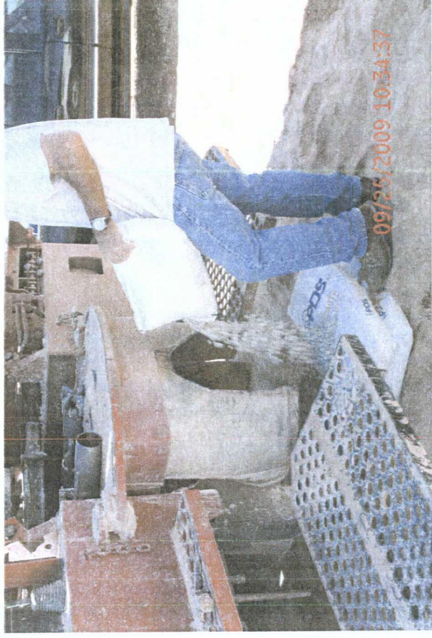
plugging SB #1 with bentonite
