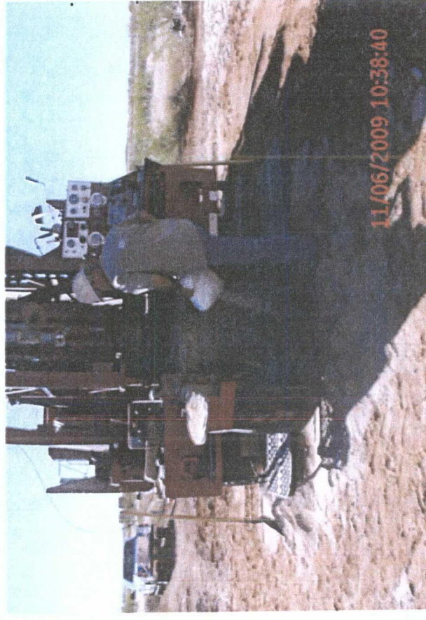
Plugging bore hole with bentonite
