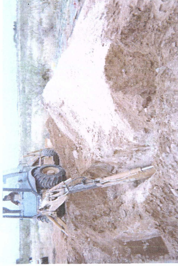
Delineation trench being excavated
