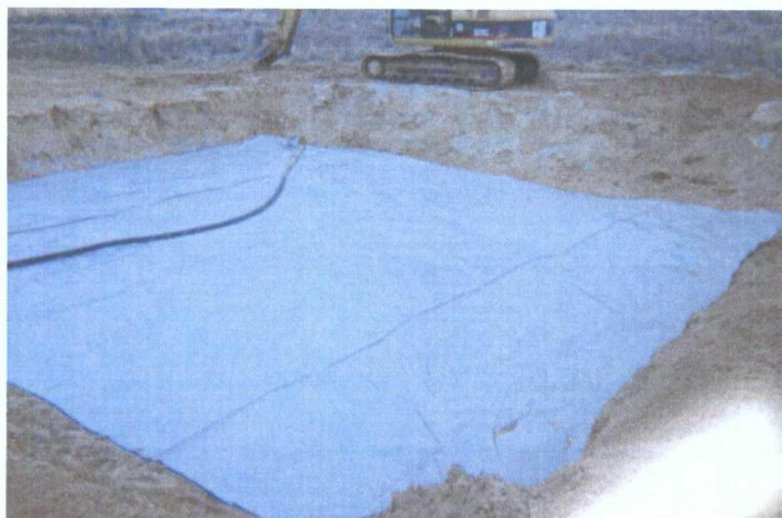
Placement of the liner
