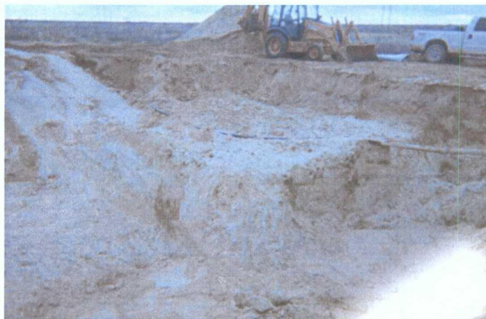
Final excavation to 5 ft BGS and 12 ft BGS on the North and East portion of the site
