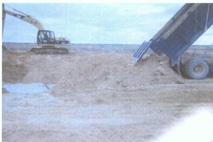
Backfilling the site
