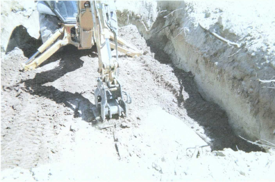
Figure 5 – Installation of subsurface clay barrier at EME N-18 Jct.
