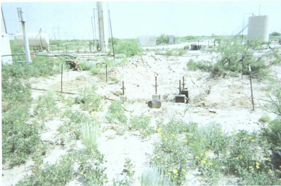
Figure 3 – Initial excavation during replacement of junction box at EME N-18.
