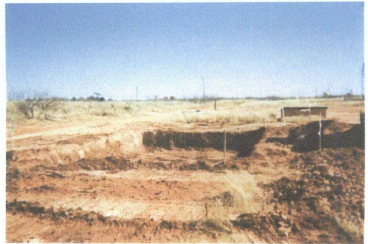
Completed excavation (22' X 28' X 4')
