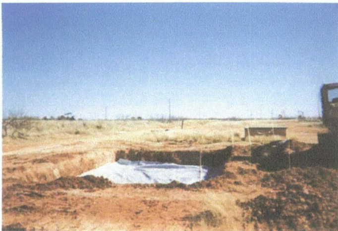
Placement of the liner in the excavation
