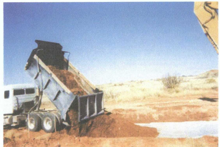
Backfilling the site with clean imported soil.
