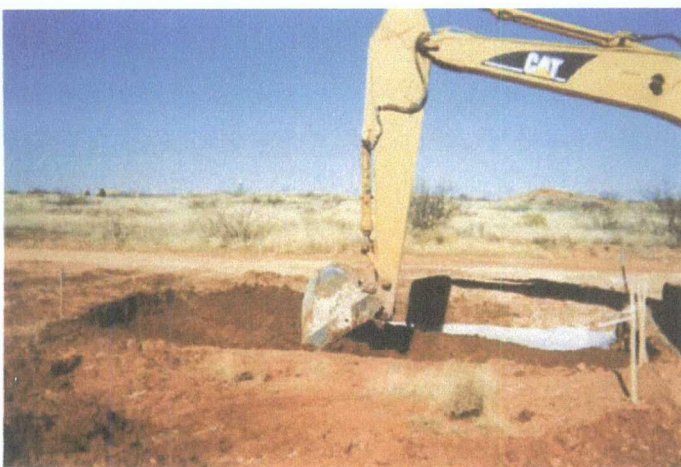
Backfilling the site with the imported soil
