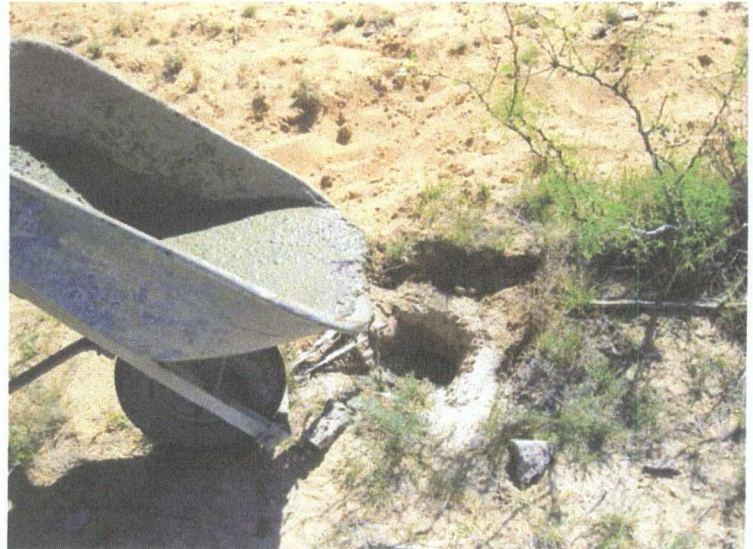
Plugging well bore with concrete/bentonite slurry
