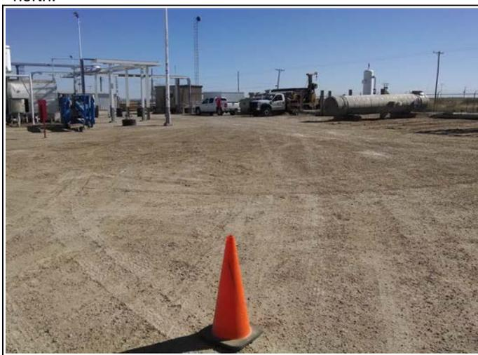
4.) View of soil boring B-18 location (at the cone), located north of the former tank battery and excavation, looking southeast.
