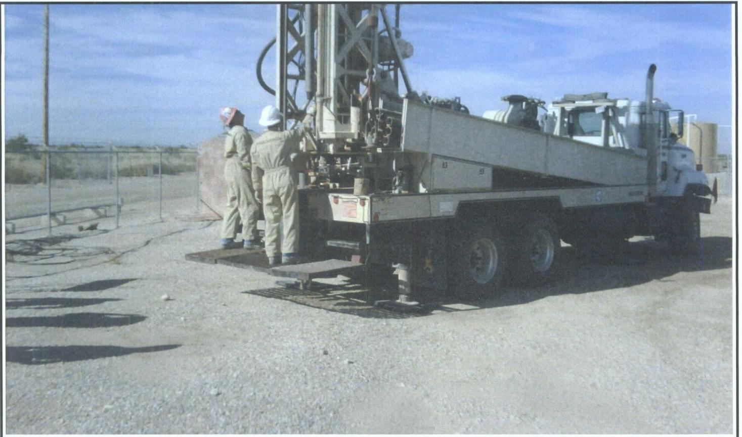
1.) Representative view of the advancement of soil boring B-1, in the vicinity of the former partially buried liquids storage tank.
