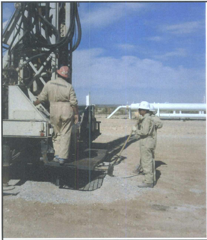
1.) Representative view of the installation of soil boring B-1.
