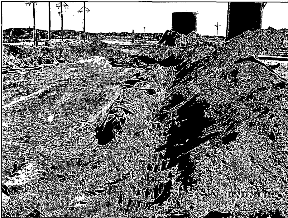
Photo 8: View of the trench for folding back the near surface sections of the primary and secondary liners. Note the near completion of the filling of the cell.
