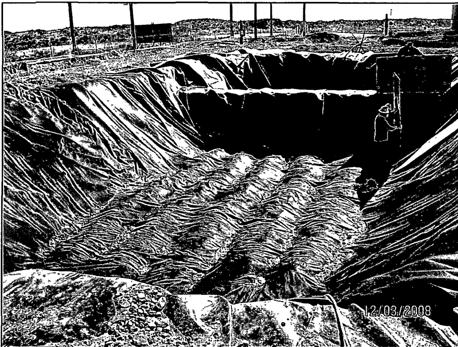
Photo 4: View with secondary 40 mil polyethylene liner, filter rock, and geotextile membrane in place. Cell is ready to wash soil.
