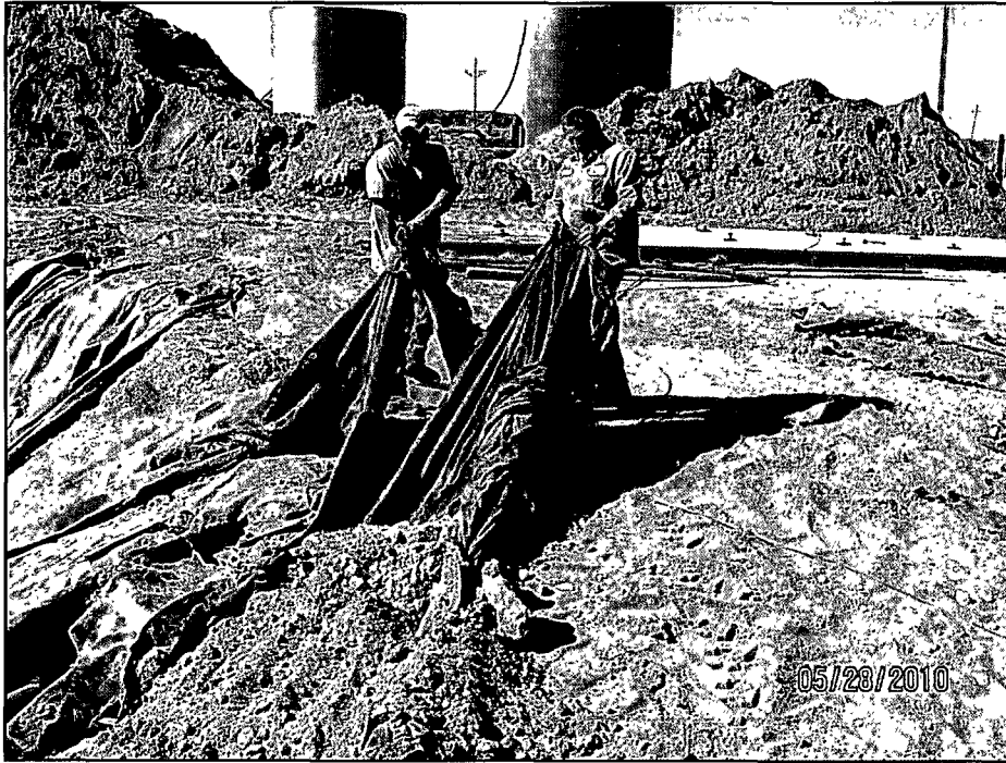
Photo 7: View of the removal of the geotextile fabric in progress.
