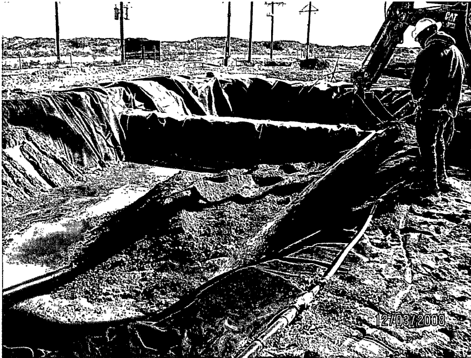
Photo 5 : Soil and water are being added to the washing side of the treatment cell.
