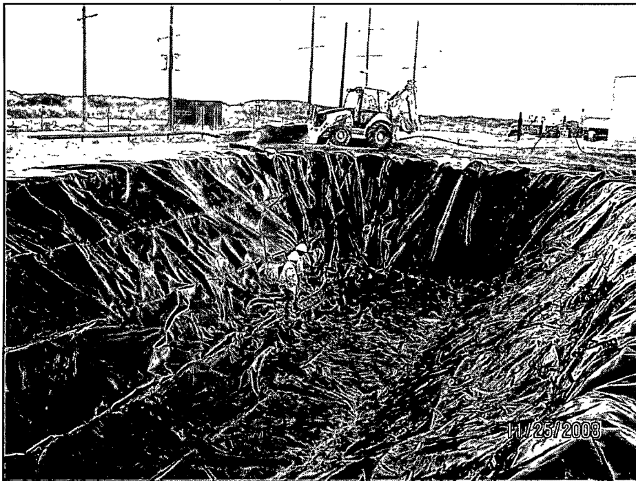
Photo 2: View of the cell following the installation of the primary, 40 mil polyethylene liner.
