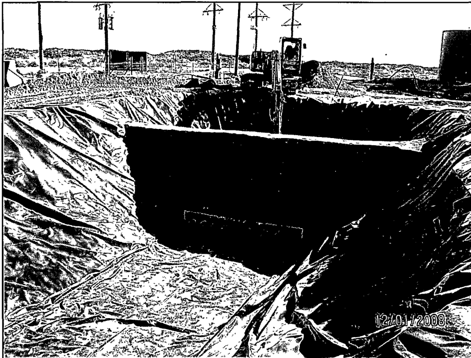
Photo 3: View of the completed divider wall to allow washing and the collection of rinsate.
