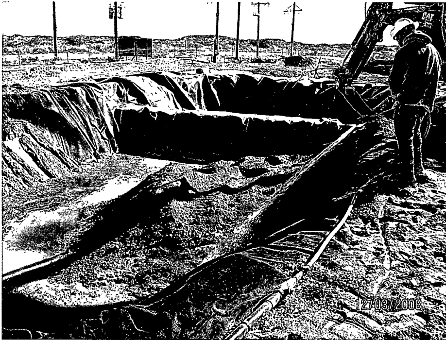
Photo 5 : Soil and water are being added to the washing side of the treatment cell.
