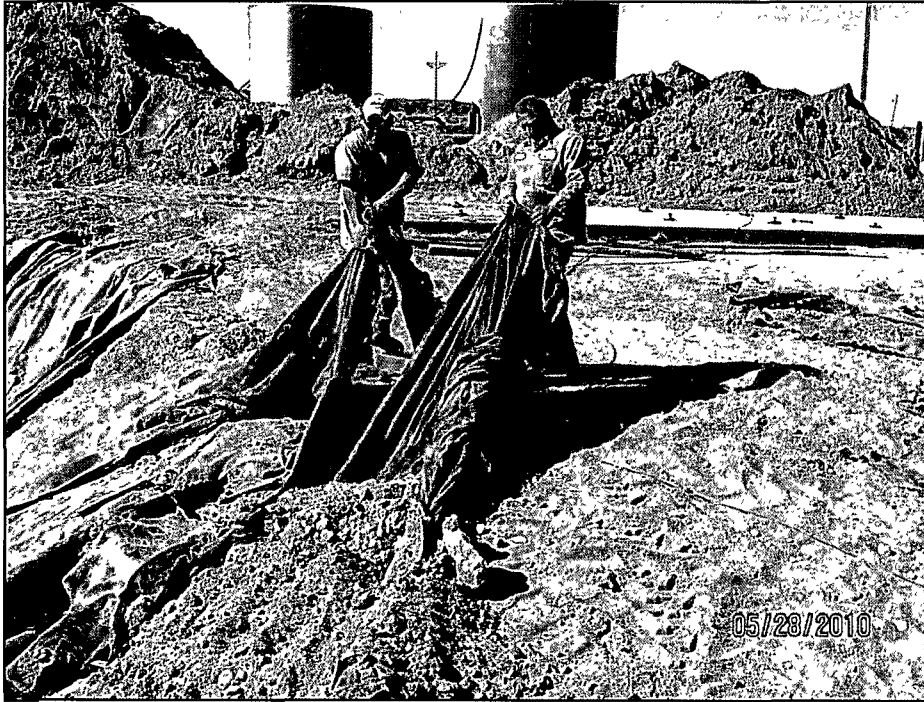
Photo 7: View of the removal of the geotextile fabric in progress.
