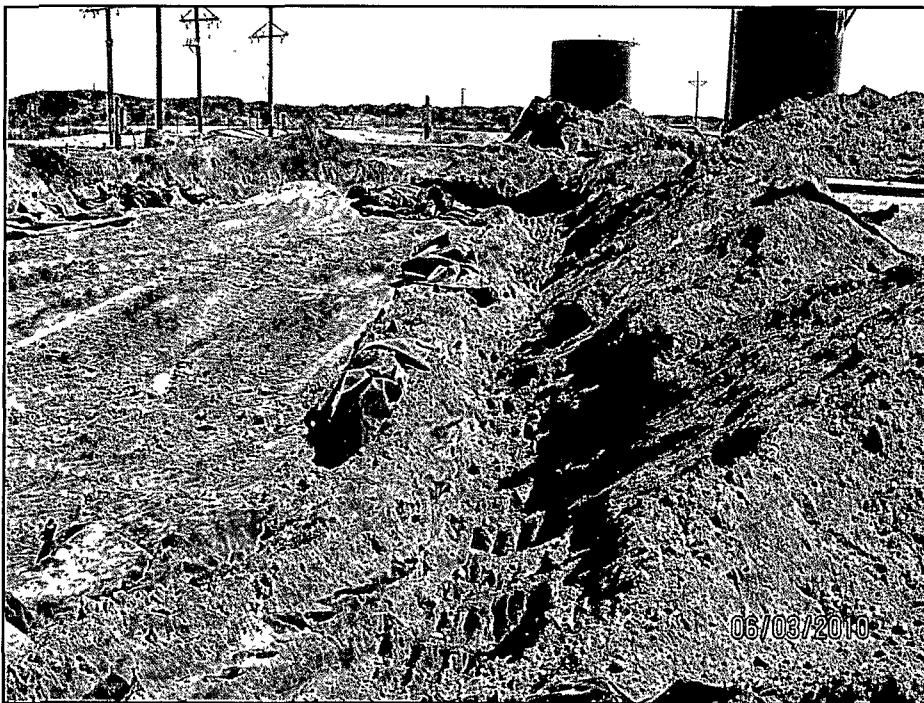
Photo 8: View of the trench for folding back the near surface sections of the primary and secondary liners. Note the near completion of the filling of the cell.
