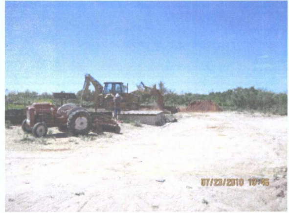
spreading top soil blended with hay
