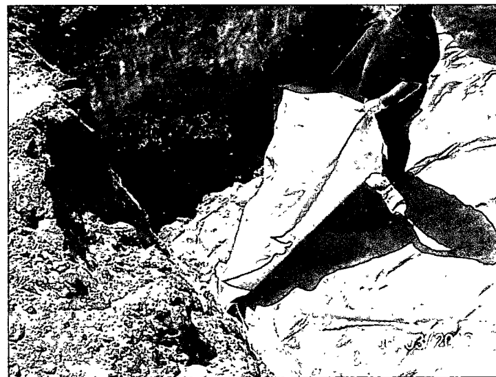
blow sand padding beneath the 20-mil poly liner
