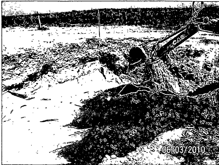
blow sand padding above the 20-mil poly liner
