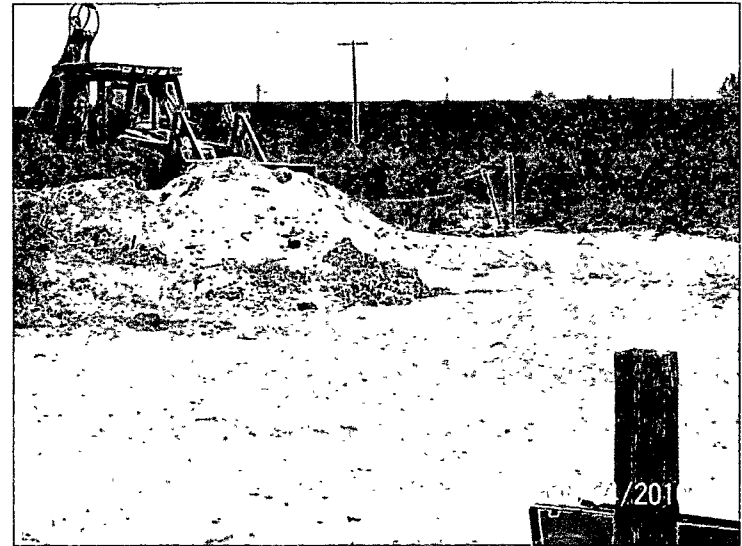
blending clean, imported soil with hay to be utilized as backfill
