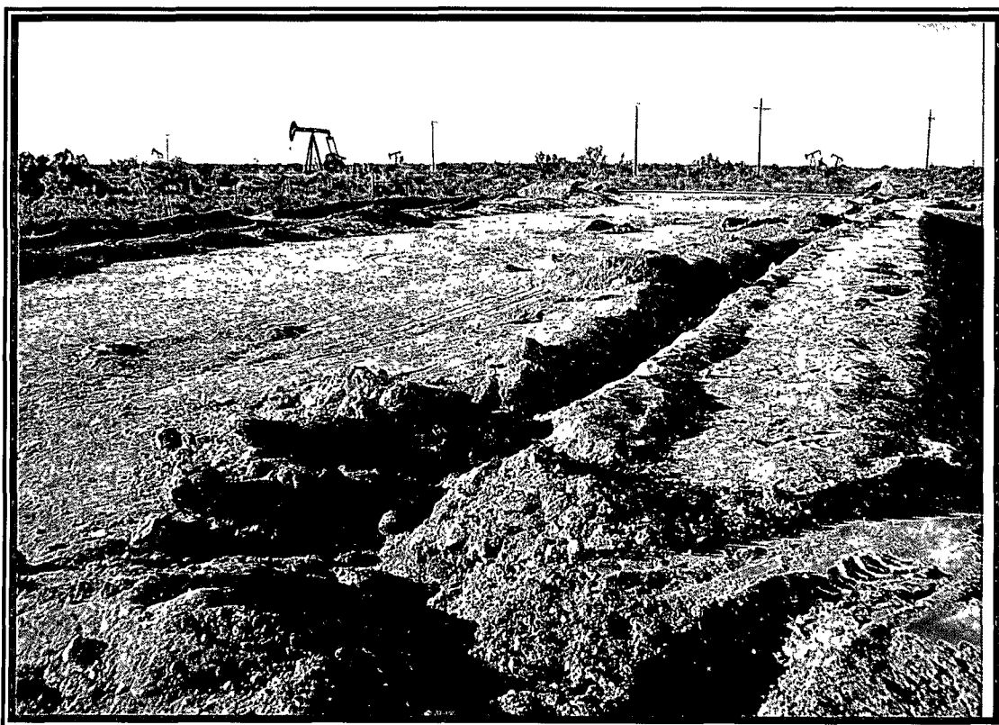
#6 Retaining trench used to hold liner edges
