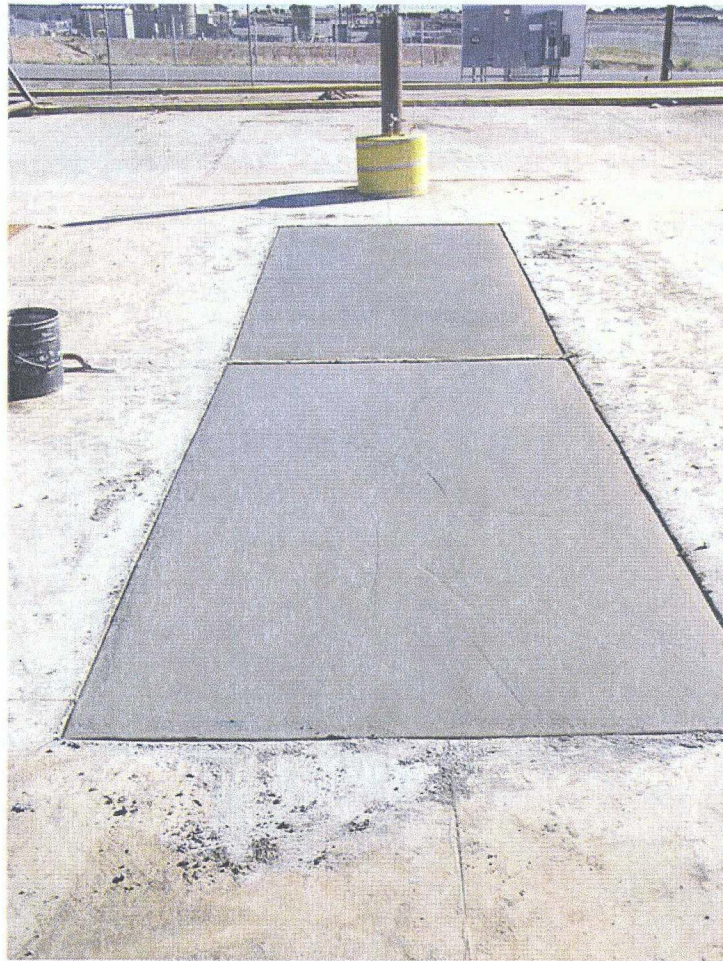
Finished concrete over sumps
