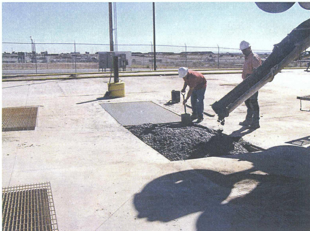
Both sumps being filled with concrete during closure activities
