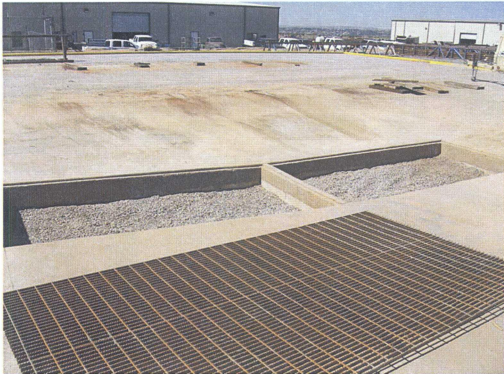
Sumps partially filled with gravel
