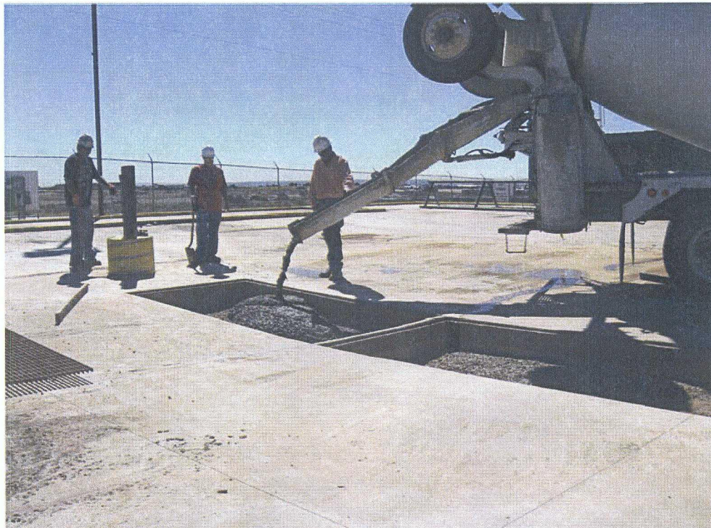
Sump partially filled with gravel
