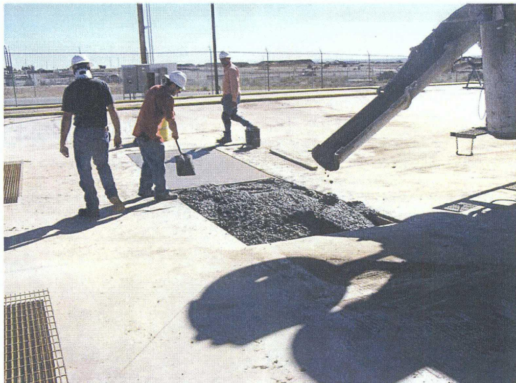
Filling the west sump with concrete
