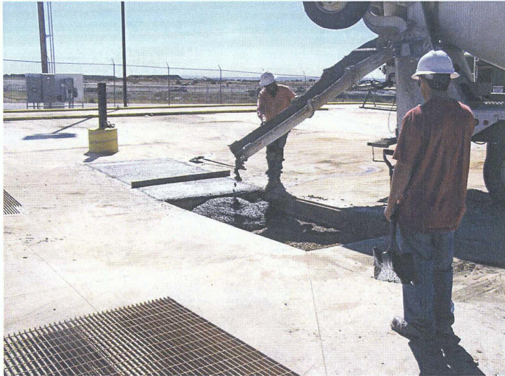
Filling the sumps with concrete
