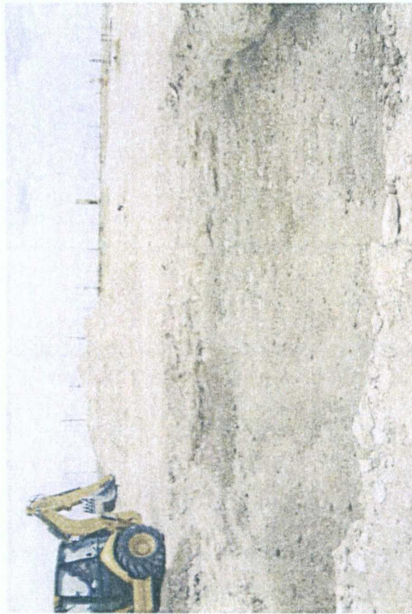
site backfilled up to 4' BGS in preparation for GCL 3/26/2008
