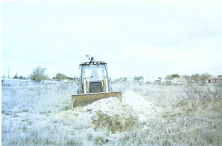
Backfilling trench
