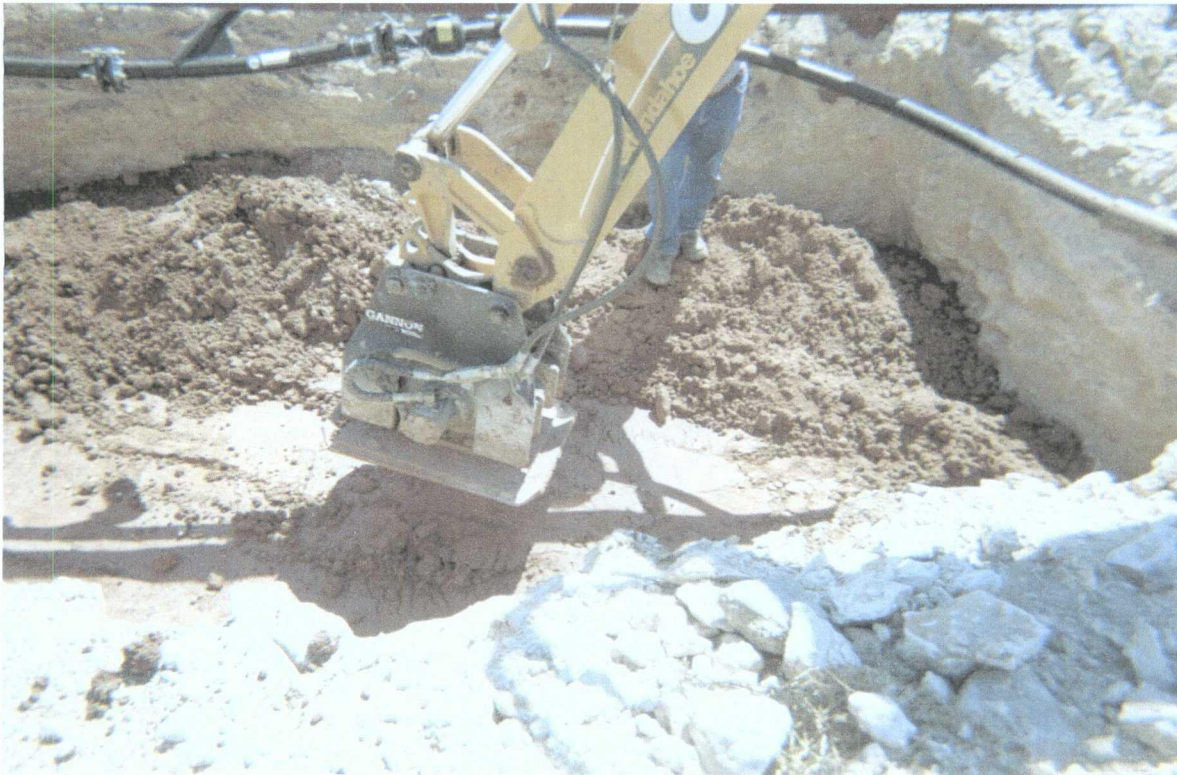
Figure 9 – Installation of clay infiltration barrier installed beneath affected area in September 2004.
