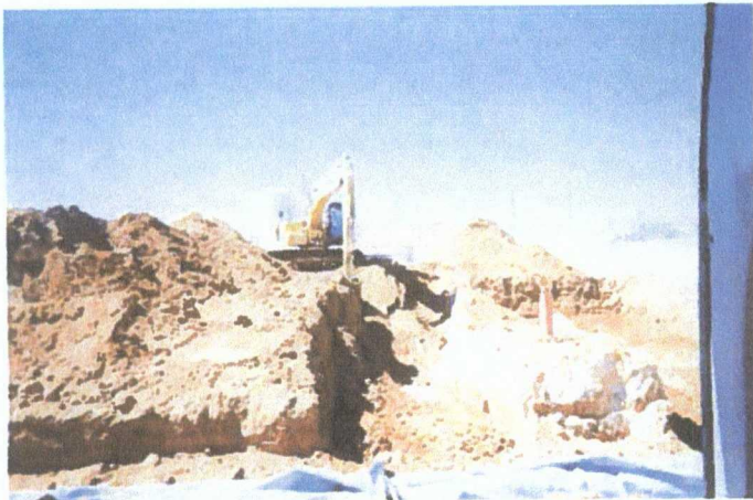
Excavating BD K-4 leak to 4' bgs
