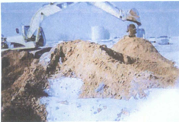
Backfilling the site with clean topsoil
