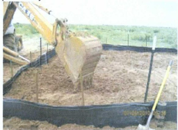
spreading clean, imported soil blended with peanut hay and amendments
