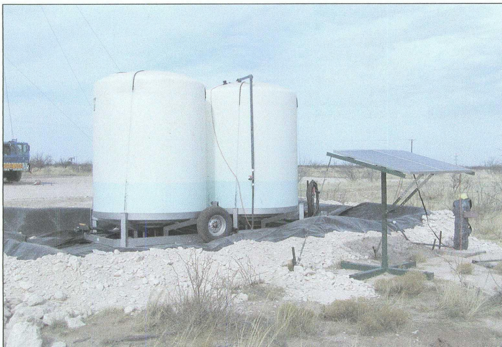
Figure 3 – Vac N-6-1 solar-powered groundwater recovery system.
