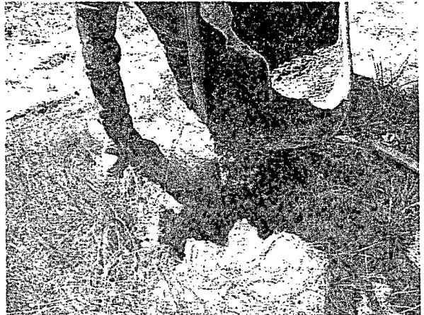
Plugging the well with 1-3% bentonite/concrete slurry
