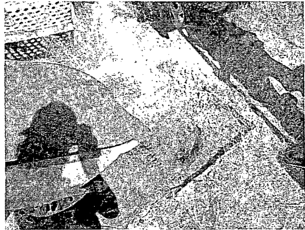
Plugging the well with 1-3% bentonite/concrete slurry
