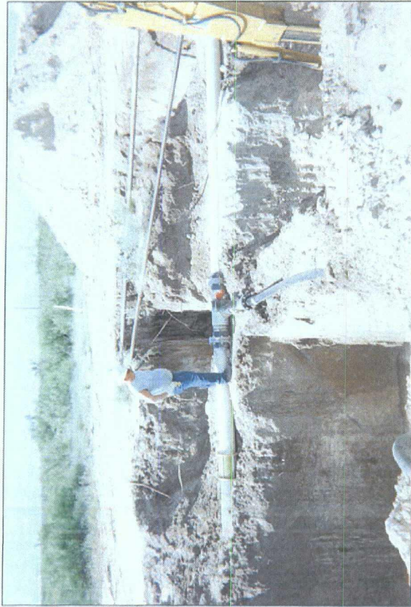
30 x 30 x 12-ft excavation with pipe supports
