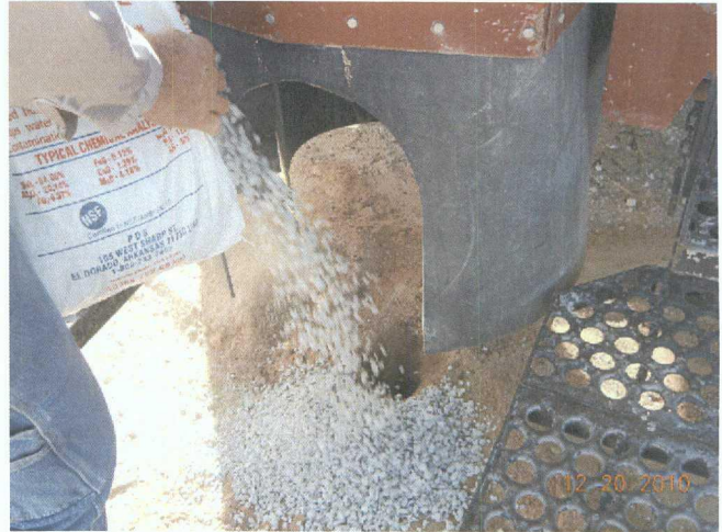
Plugging the soil bore in total with bentonite
