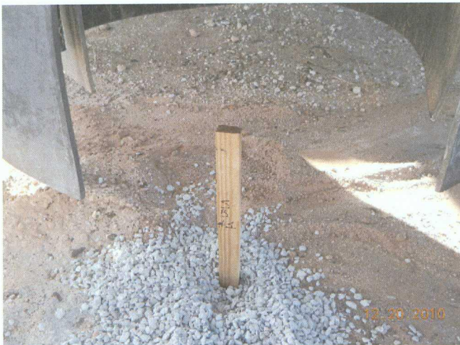
Completed soil bore
