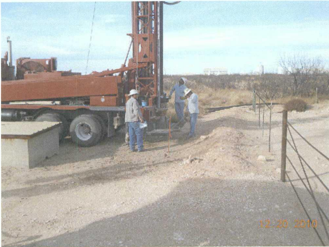
Drilling the soil bores
