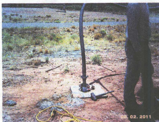
Pressure hose connected to well
