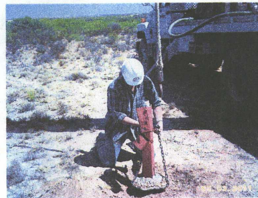
Wellhead protector removal
