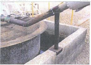
Photo 13: Fluids in secondary containment.
