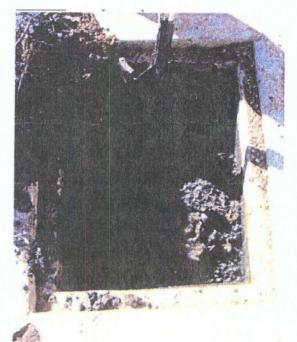
Photo 3: No drainage within sump.
