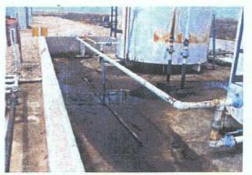
Photo 15: Fluids in secondary containment area.
