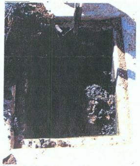
Photo 3: No drainage within sump.
