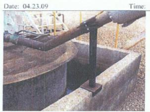
Photo 13: Fluids in secondary containment.
