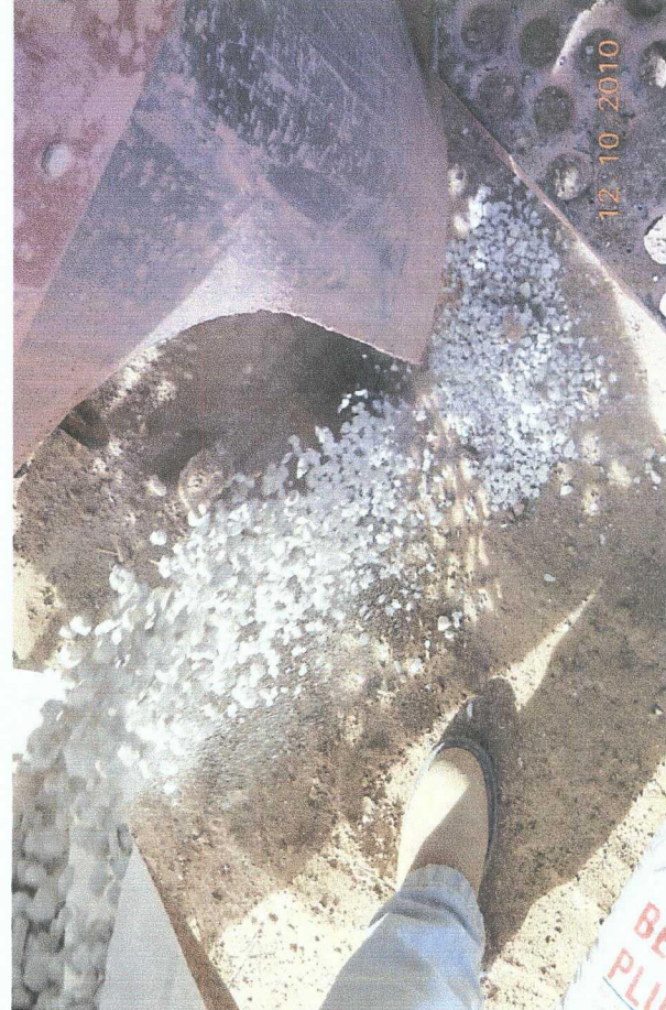
Plugging bore hole with bentonite
