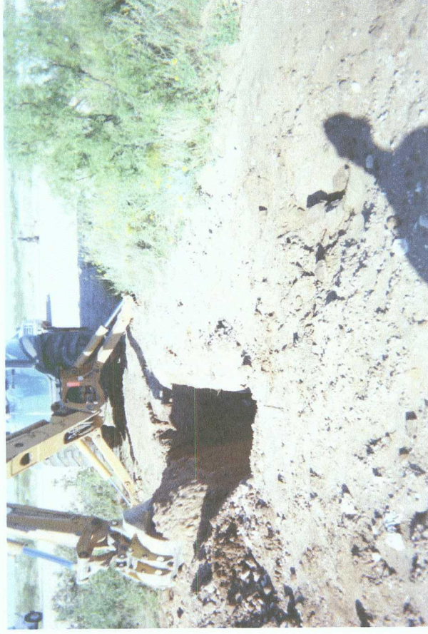
Backfilling trench
